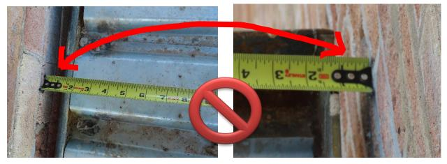
Extra care must be taken to make sure that the opening is the correct size and parallel
